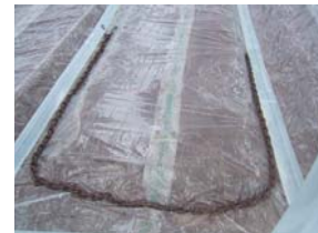
④ Completed preparation.
